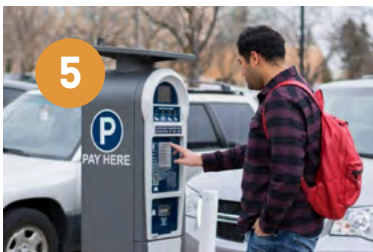
Revenue Control Equipment: Installing devices and software used to manage and collect revenue from parking facilities, such as meters, pay stations, and ticket dispensers
